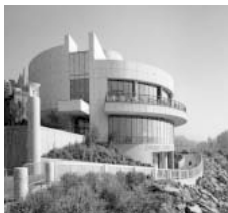
Foto 1 - Boathouse em Sawyer Point, Cincinnati, Ohio (PCI, 1989).
